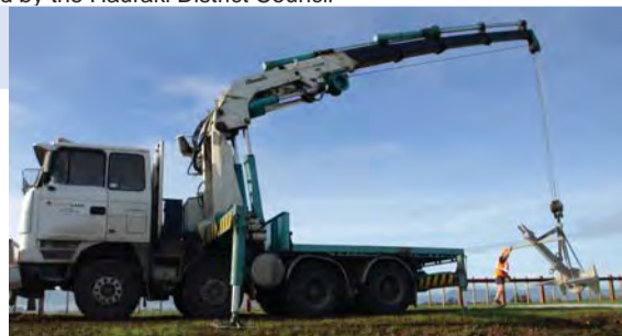
Above: Mike Smith of HydraCare Thames guides the anchor into position
