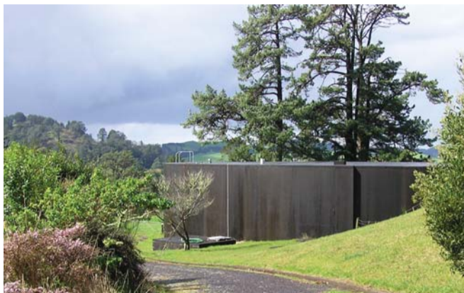
Above: The Waihi Water Treatment Plant
