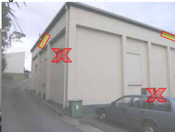
Figure 2: North Wall west corner
