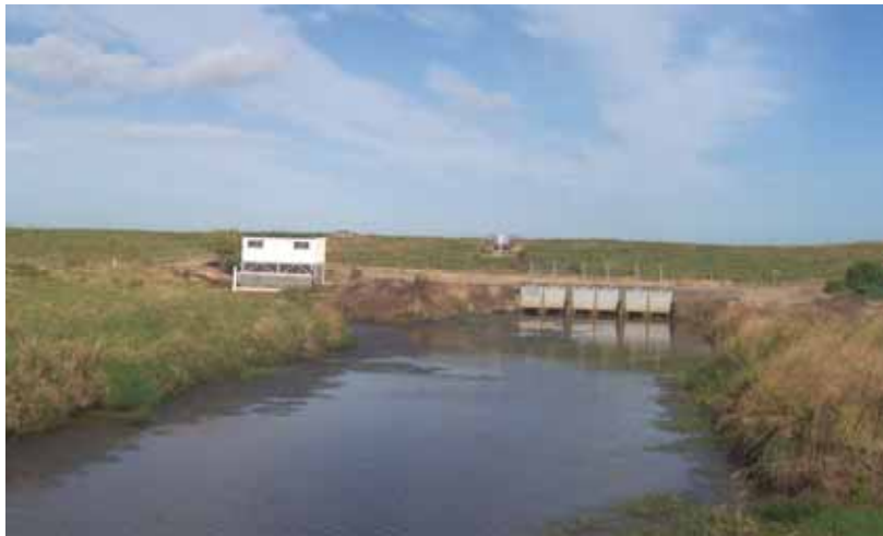
Tirohia Canal, Mill Road Pump Station and Floodgate
