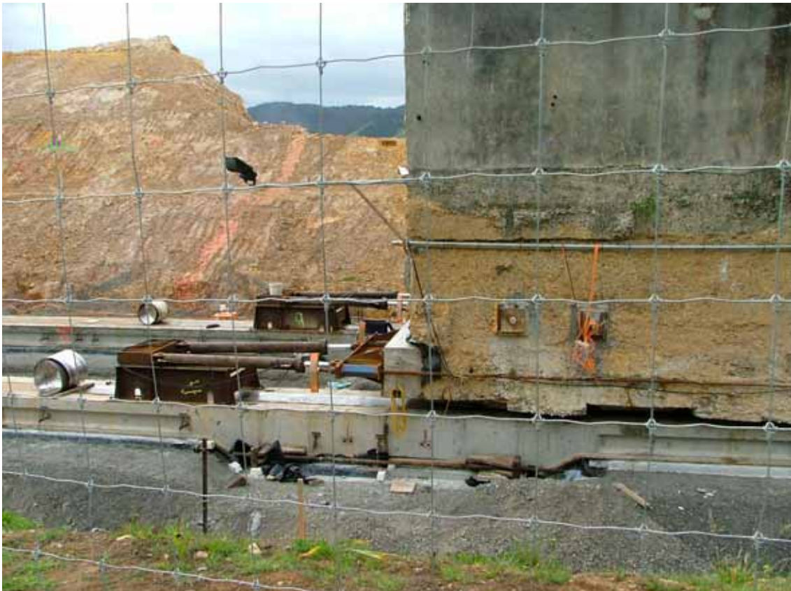
Frontispiece The iconic Cornish Pumphouse on the move past the end of Gilmour St. to site 4A, late October 2006
