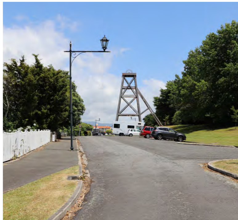
Poppet Head: view looking south west towards Seddon Street.
