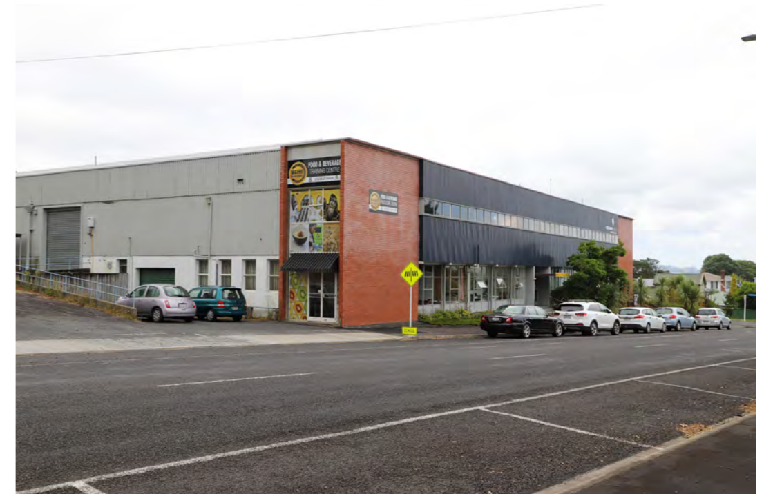
Pye Building: view looking south east from Moresby Street.
