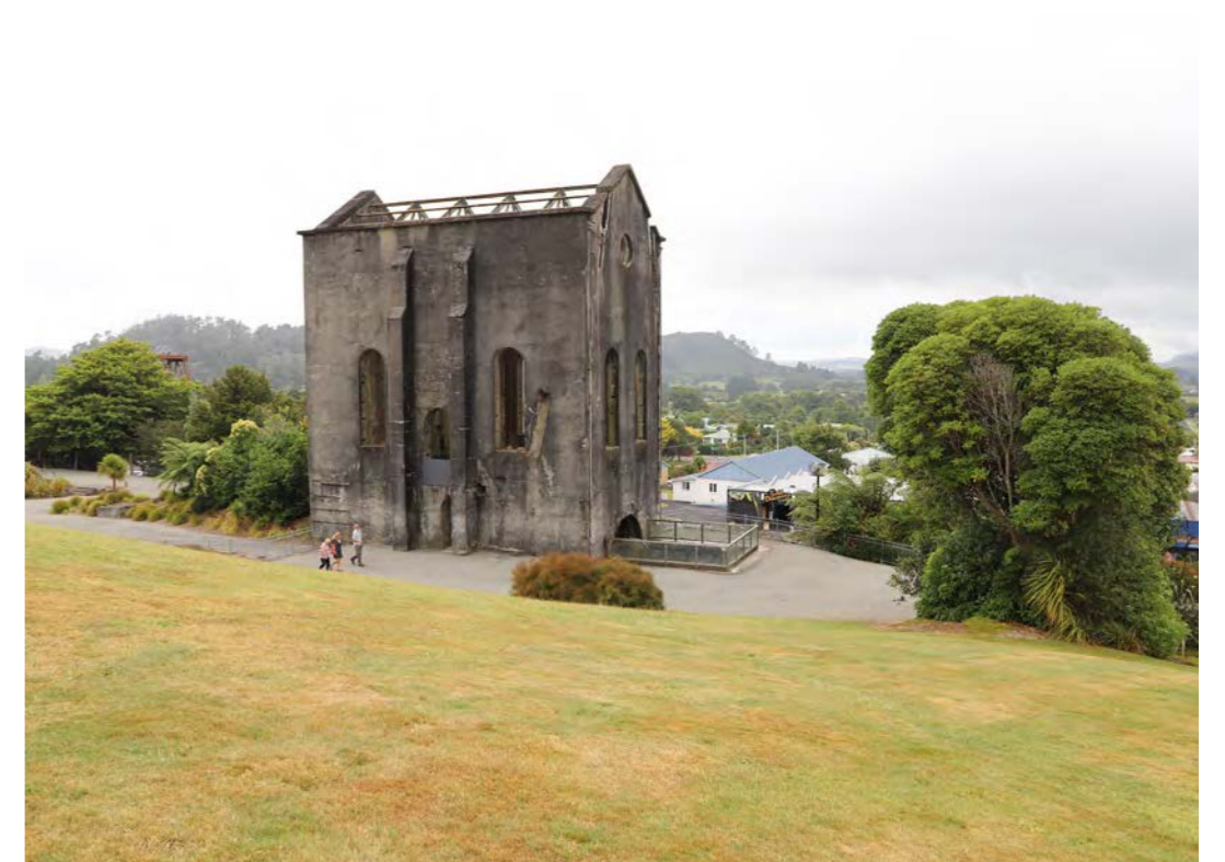
Pumphouse: view looking south towards the Pumphouse with the Poppet Head in the distance.
