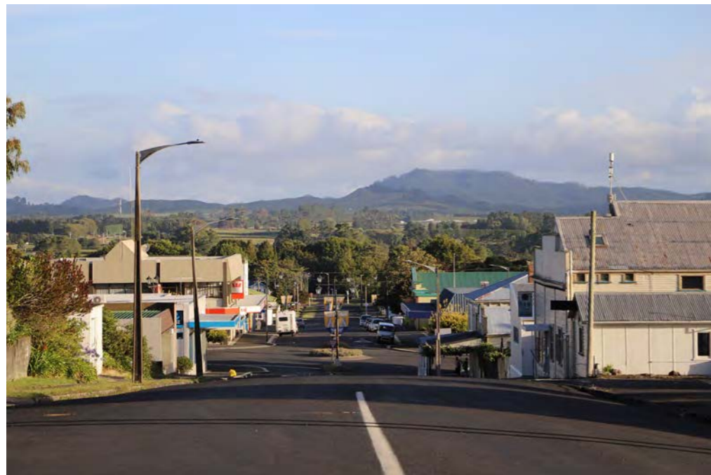
Hazard Street: view looking south east towards Seddon Street roundabout.
