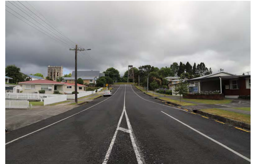
Gilmour Street: view looking north along towards the Poppet Head.
