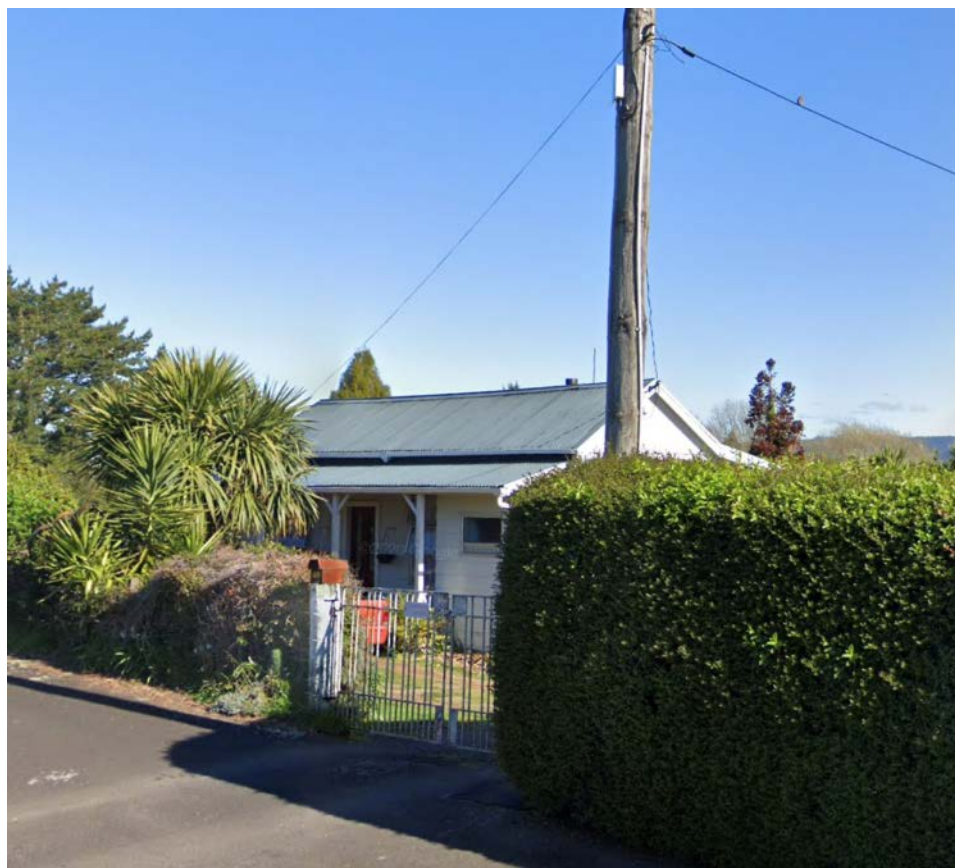
Figure 30. Early 20 th century cottage at 48 Moresby Avenue
