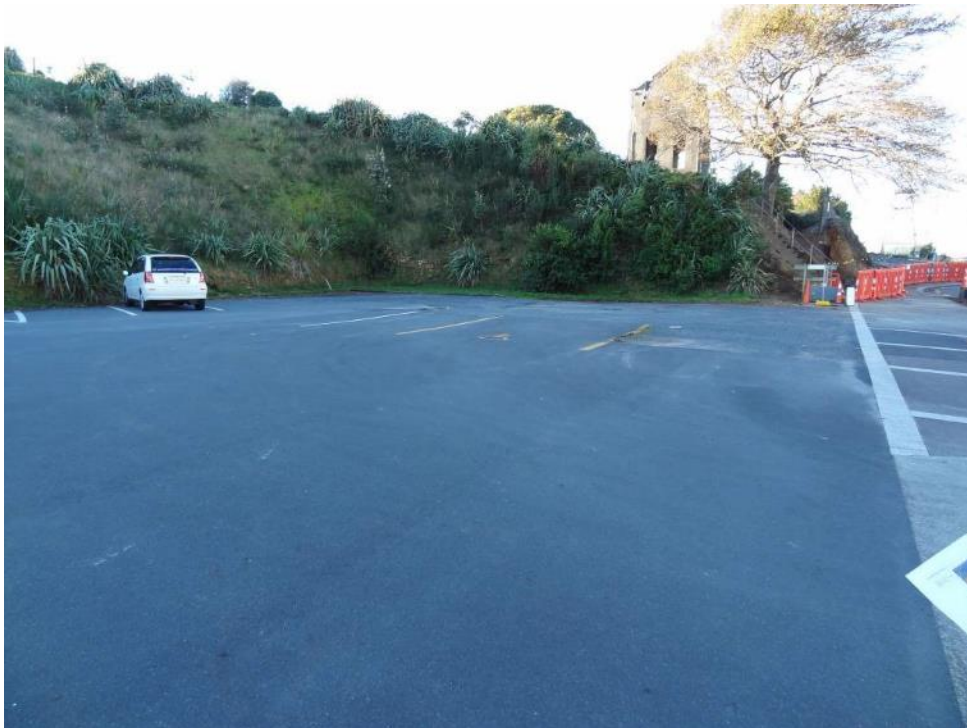
Figure 44. The cut back and battered slopes behind the carpark on 73-75 Seddon Street looking east towards the Pumphouse
