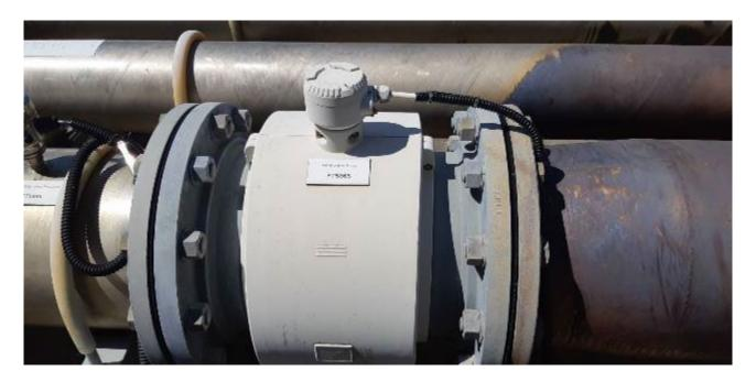
Figure 3: Dewatering totalising flow meter
