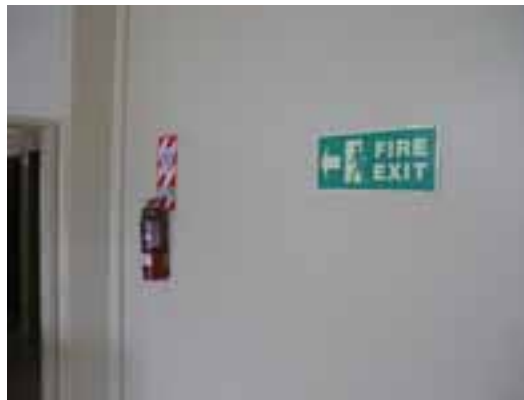
Kitchen Fire Extinguisher
