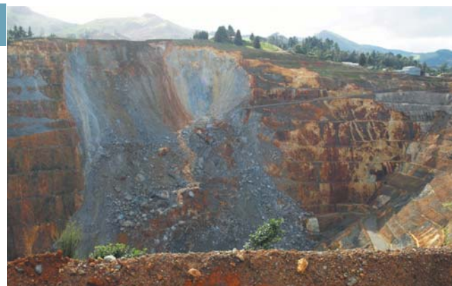
SLIPPERY SLOPE: Heavy rain has acted as a lubricant on the failed north east wall of the Martha pit.
