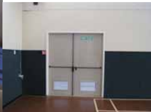
South Wall Exit
