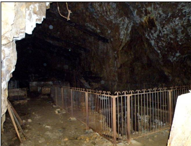
Pumphouse interior 2010 with some ceiling timber still in place.
