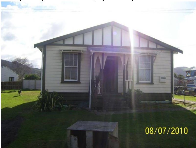
Railway Factory House Built 1925, Style: roof D porch D
