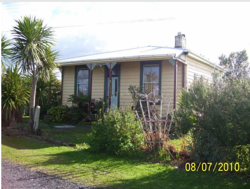
Platelayer Cottage Built 1906; Design referred to as a 'sunshine house'; Class B public works design (Mackay 1994:13).
