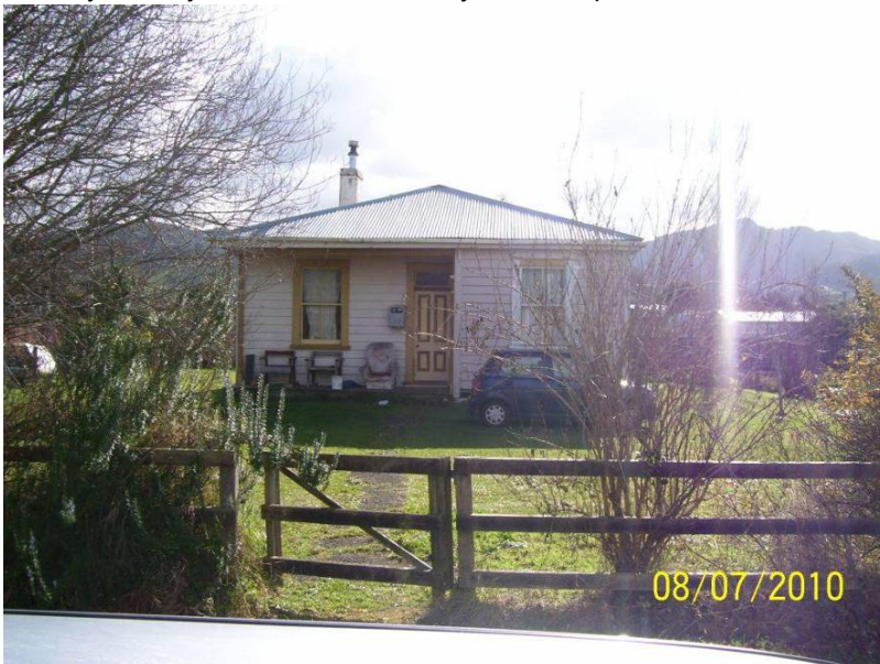
Platelayers Cottage, Built 1904/05.
