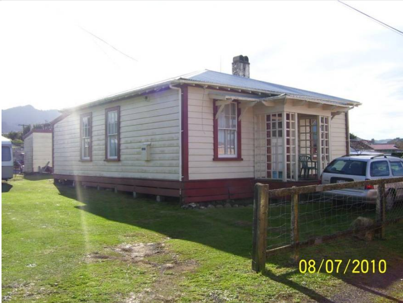
Railway Factory House Built 1925, Style: roof C porch C
