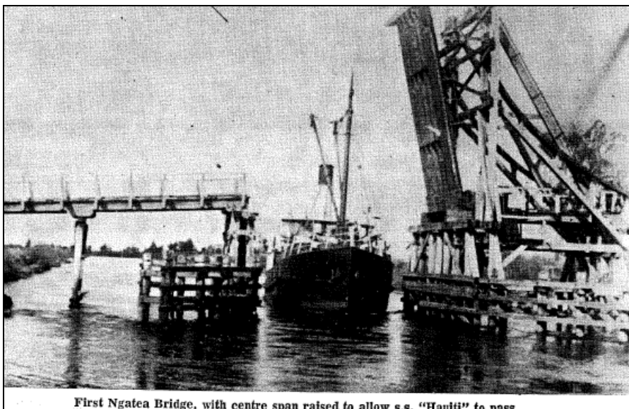
First Ngatea Bridge, with centre span raised to allow s.s. "Hauti" to pass.
