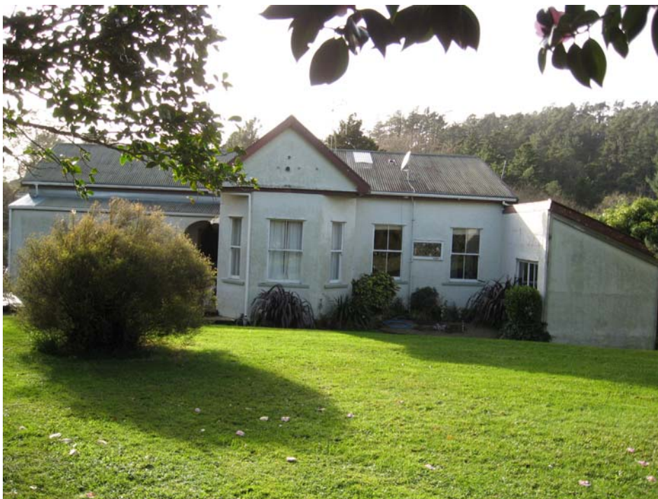
Rear Elevation of the Battery Manager's House at 10 Baker Street, 2011
