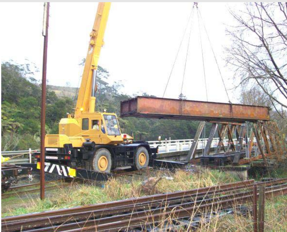
Waitekauri Bridge, Maintenance Work (The Goldfields Express July-August 2010:3 www.waihirail.co.nz )
