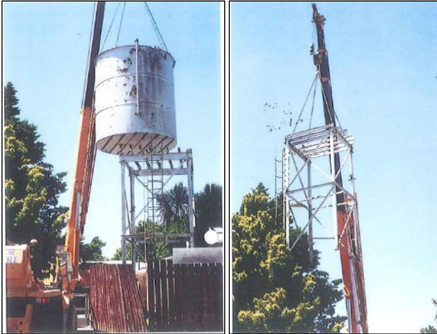
Removing water tank and stand
