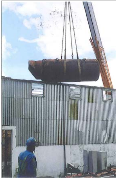
Boiler being lifted out of No. 2 Boiler Room
