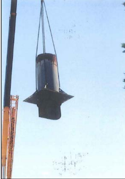
Lifting chimney base
