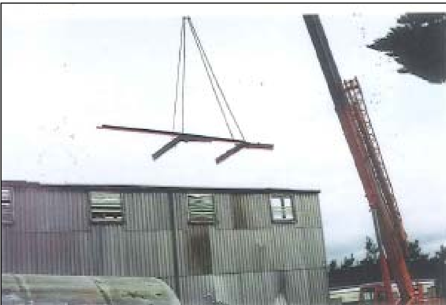
Roof frame off No. 2 Boiler Room
