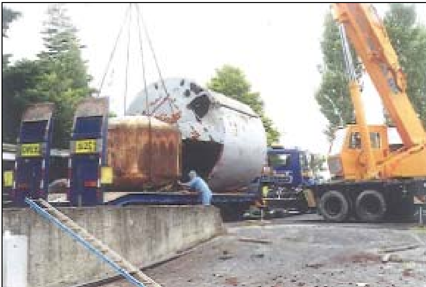
Water filter and tank ready for removal on transporter
