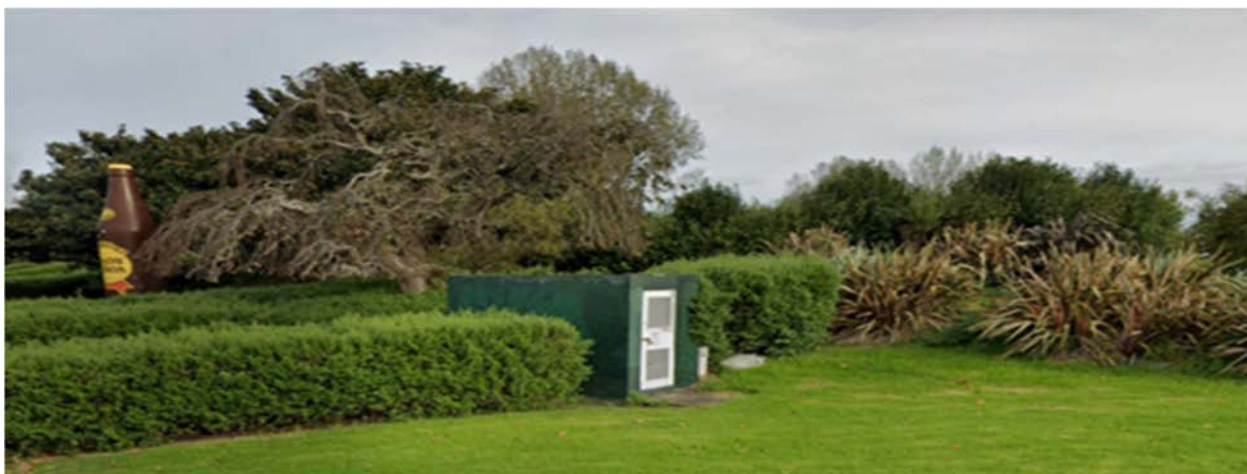
Criterion Bridge Pump Station
