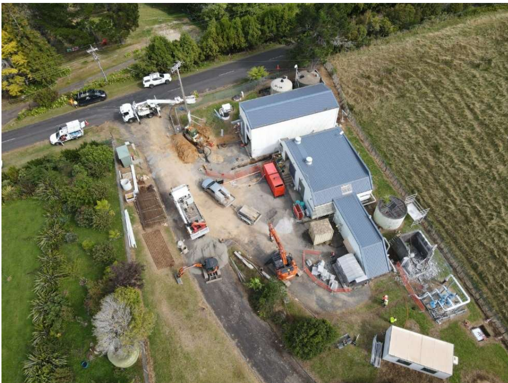
Transformer location work underway
