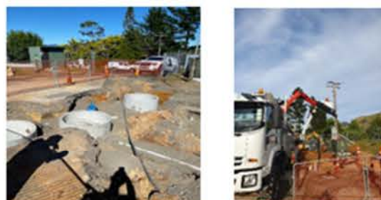
Manhole installation for storm water and wastewater
