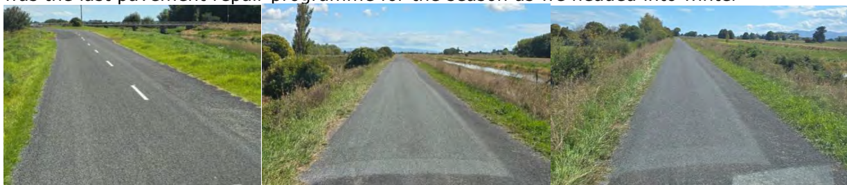
Image 8, 9 & 10 – Pavement repairs around the network
