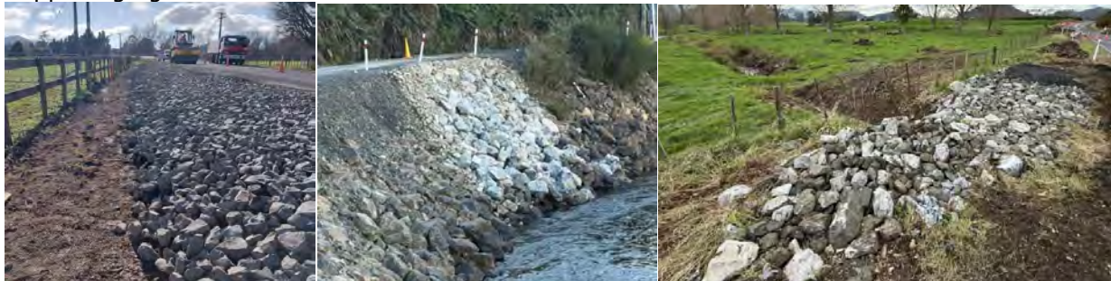
Image 5, 6 & 7 – Frankton, Franklin & Crean Road – Washout repairs from 20 th January storm event.
