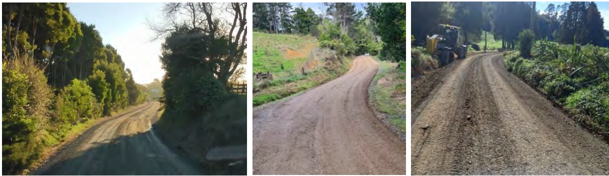
Image 15, 16 & 17: Spot metalling works.
