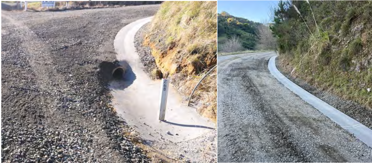
Image 11 & 12 – New surface water channel on Ngatitangata & Homunga Road, Waihi
