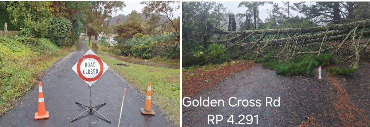
Image 1 & 2 – Flooding & damage because of cyclone Vaianu.
