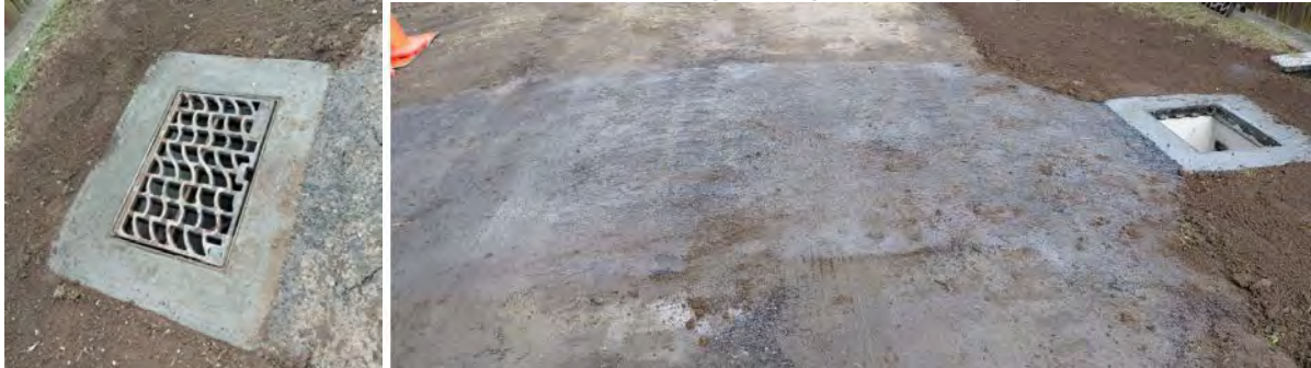
Image 13 & 14 – Catchpit & culvert renewal along River Road, Karanghake.
