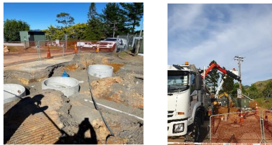
Manhole installation for storm water and w. water
