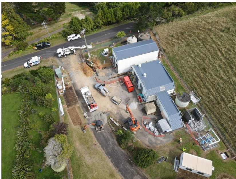
Transformer location work underway
