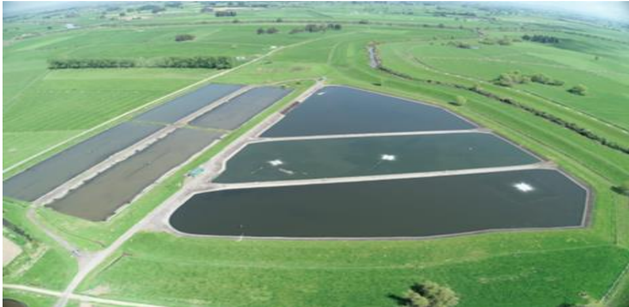
Paeroa Wastewater Treatment Plant
