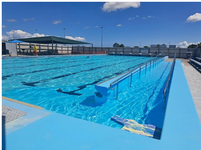
Completed Access Ramp at Ngātea Pool
