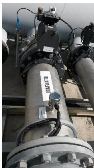
Figure 4: Underground dewatering sample spigot
