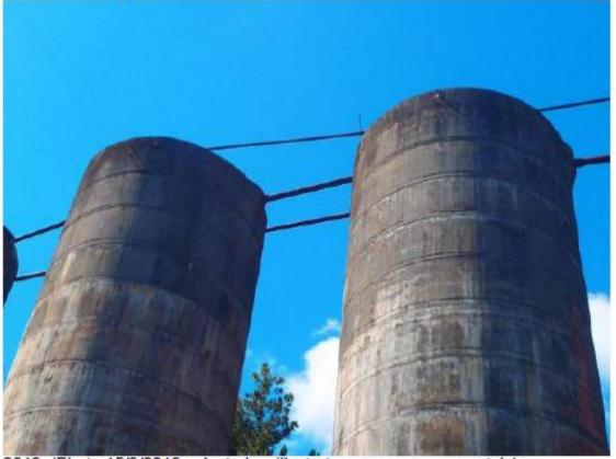
2012: (Photo 15/3/2012 selected as illustrates area more accurately) Observations: No movement evident after close examination of series. Upward projecting small pipe not moved on unrestrained length. Conclusion: No discernible change
