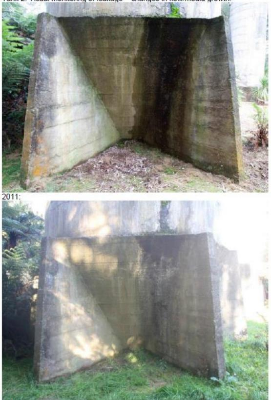
Tank 2: Visual monitoring of leakage - changes in flow/mould growth.
