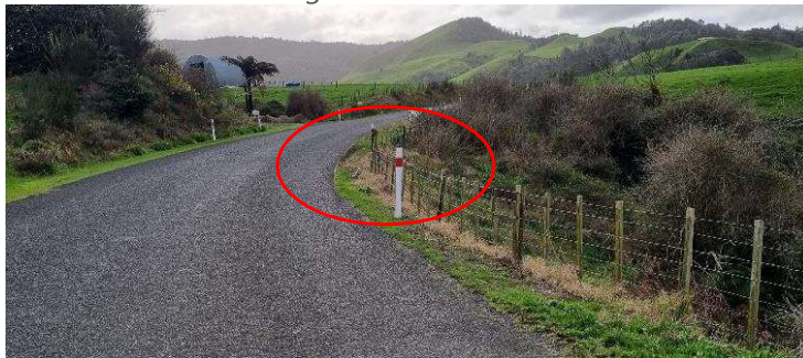
Figure 2 – Narrow & steep shoulder just south of Culvert 65, Chainage 0.62km
