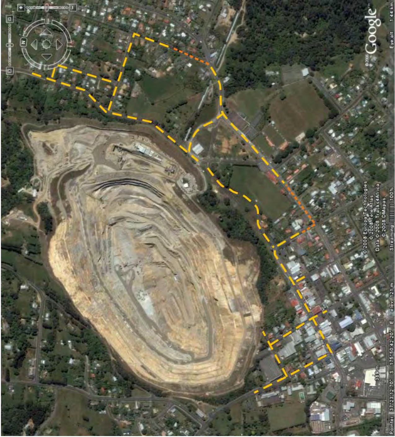
Figure 5b Yellow dashed lines show recommended monitoring lines with points at ~20m spacing and incorporating as many existing settlement monitoring points as possible (Figure 7 & 7a). Orange dashed lines are linking lines using existing points.
