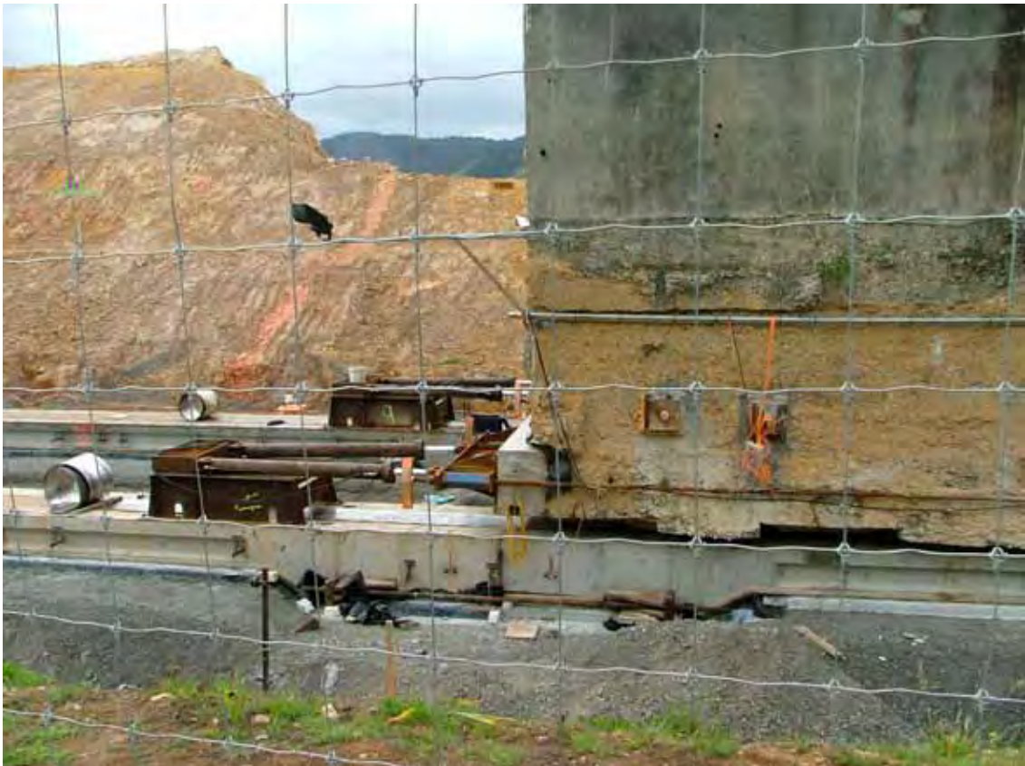
Frontispiece The iconic Cornish Pumphouse on the move past the end of Gilmour St. to site 4A, late October 2006
