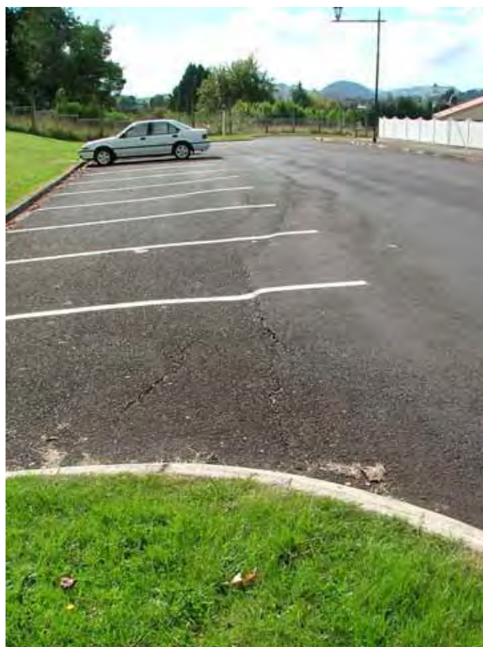
Photos 3&4 Cracking in Seddon Street appears to be extensional but also has a small right lateral component of movement in the pavement above.
