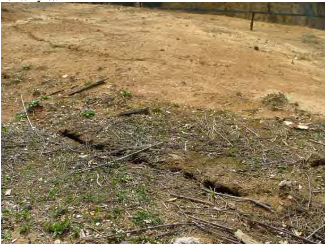
Photo 6 & 7 Open ground cracking with north (pit) side up, close to the pit rim and east of the Judges Kauri.
