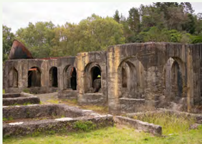
Above: Victoria Battery, Waikino
