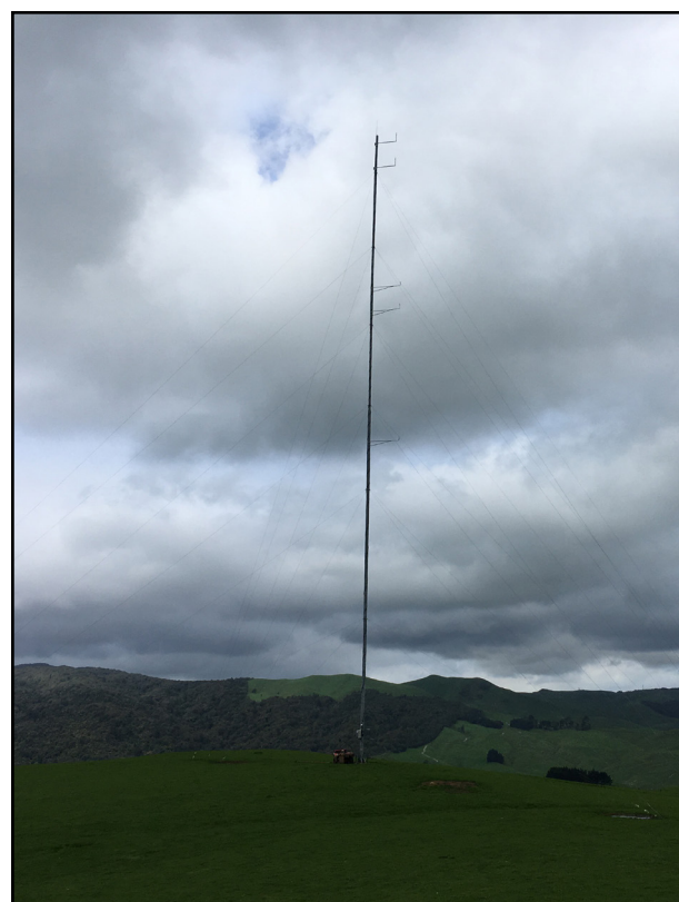
One of the monitoring masts.
