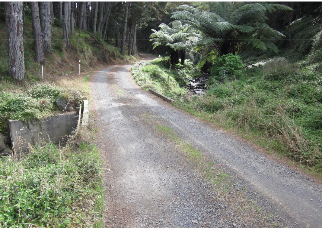
Figure 12: Existing Access Road Showing Culvert
