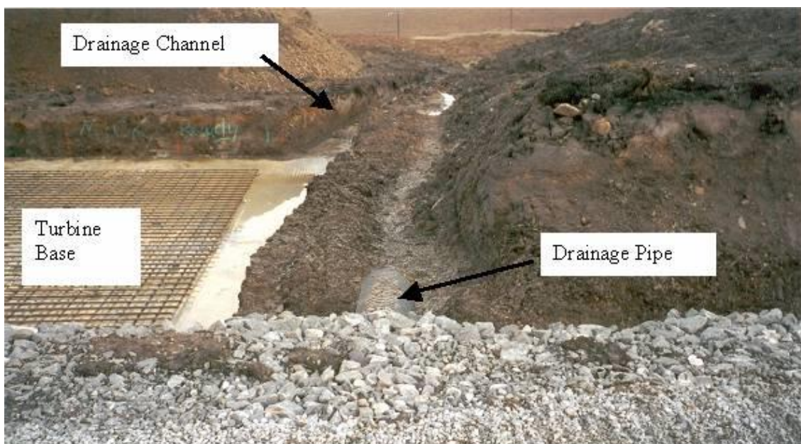
Figure 5 - Good Drainage Practice
