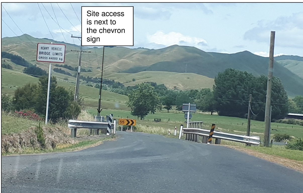
Figure 11: One lane bridge on Rawhiti Road west of the site access.
