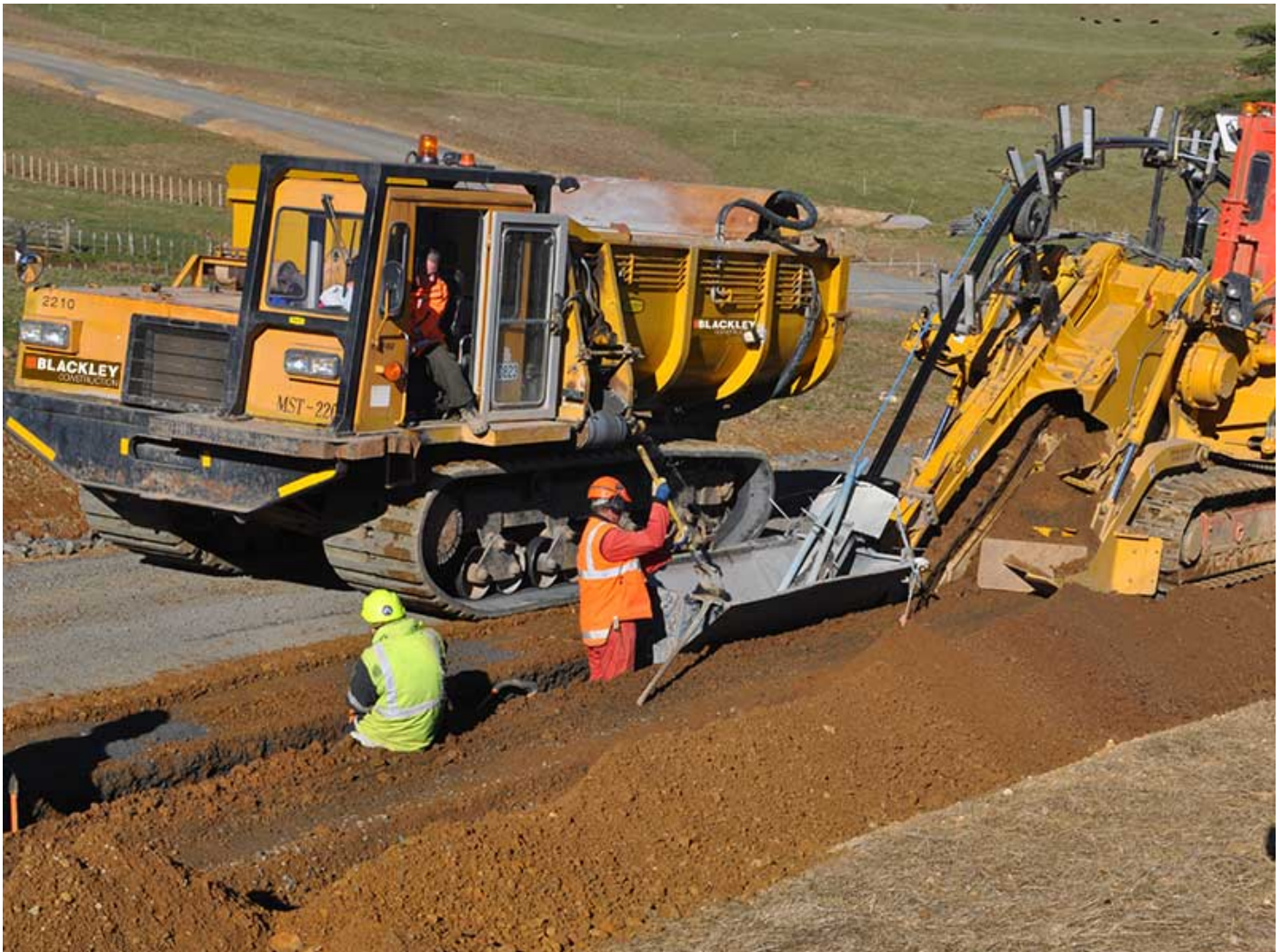
Figure 12. Cable laying Te Uku Wind Farm
