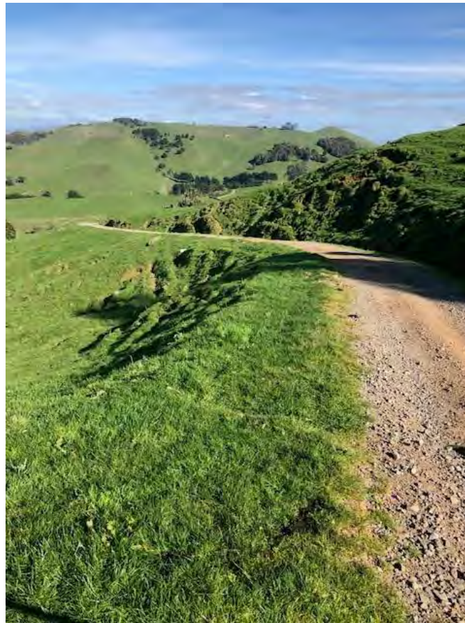
Plate 1: Existing access track formation
