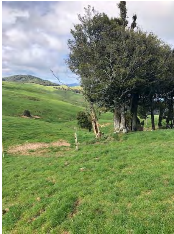
Plate 6: Fill Location Ch 3200
