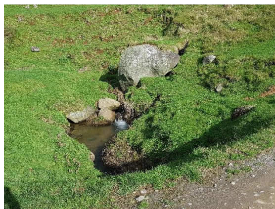
Plate 24 View of downstream of C7
