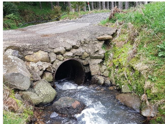
Plate 10 View of upstream looking down on C3
