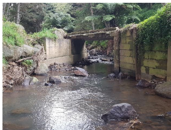
Plate 3 View of downstream looking up to C1
