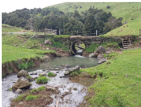
Plate 13 View of downstream looking up to C4
