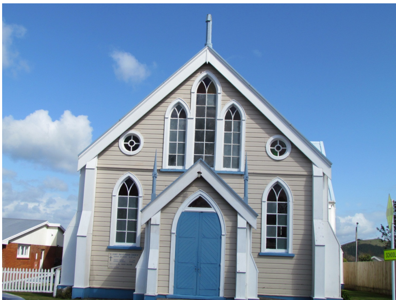
Front Elevation – Moresby Avenue Frontage Note Buttresses on corners. These do not contribute to lateral stability
