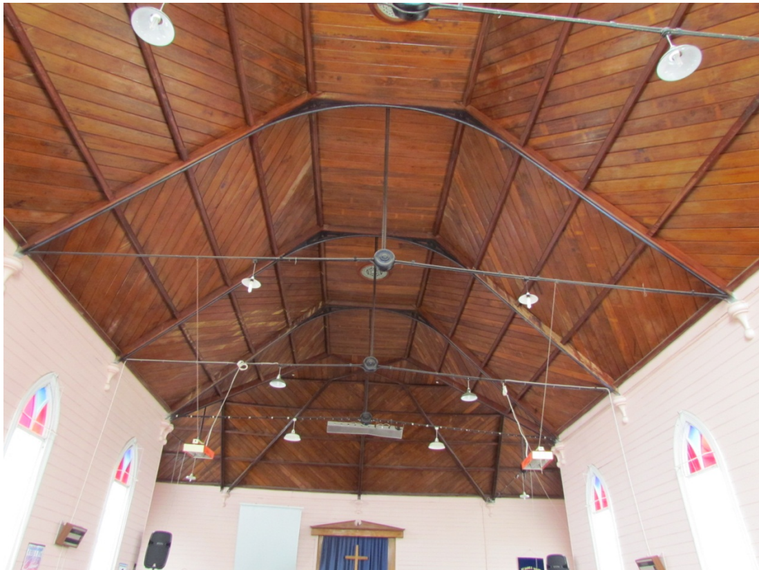
View of Nave Ceiling – Note Timber Panelling and steel rod ties between walls
