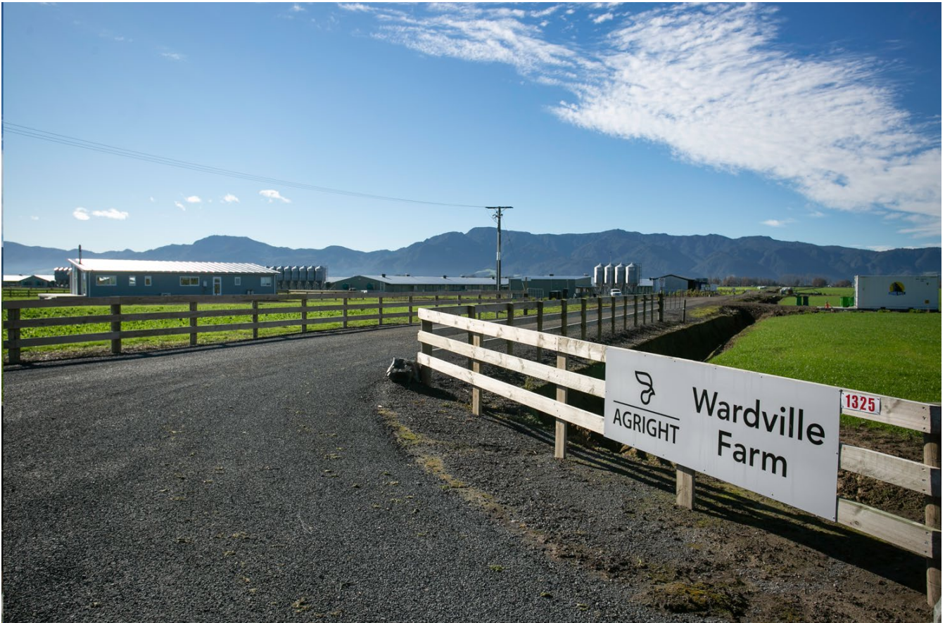
Figure 5: Example Chicken Farm (Wardville) – Photo taken from farm entry gate off Alexandra Rd
