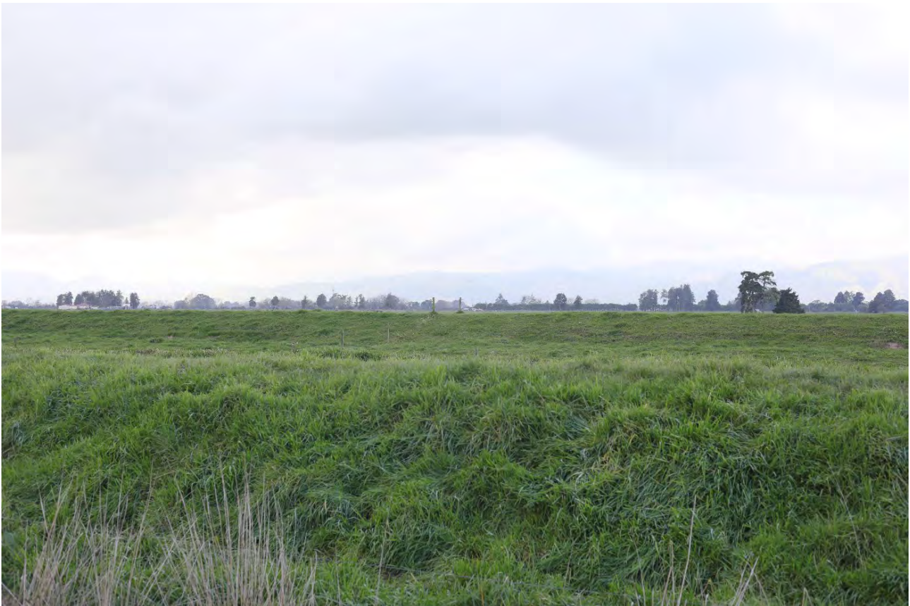
Figure 16: Grassed Awaiti Canal stop banks west of the proposed development sites.
