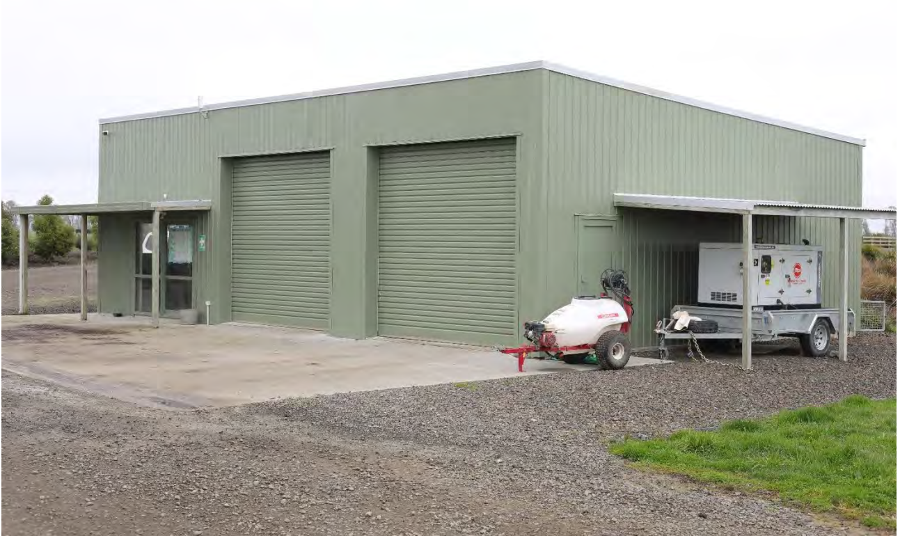
Figure 6: Wardville Broiler Farm example of machinery/storage shed.
