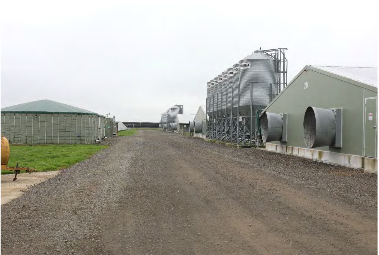
Figure 3: Wardville Broiler Farm example of poultry sheds, chicken feed silos, water tanks, machinery/storage shed and perimeter access road (similar configuration to proposed development).
