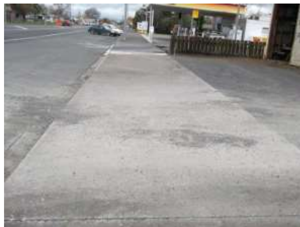
Figure 19: Entrance to Hauraki Engineering Ltd
