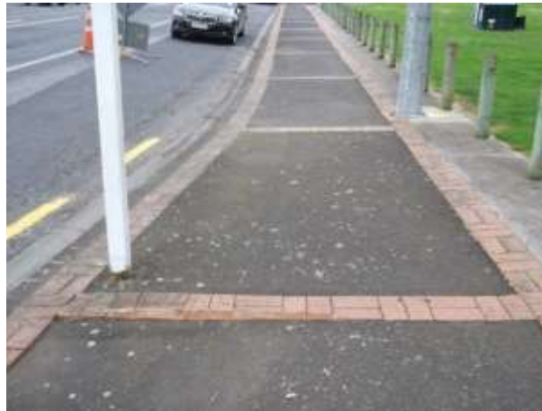
Figure 14: Footpath surface on Sh.2
