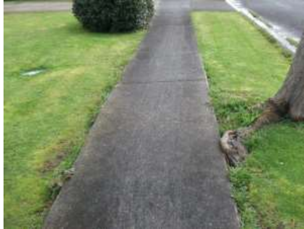
Figure 18: Tree root lifting footpath at 14 Madgwick Place
