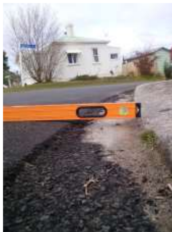
Figure 11: Seal edge join after re-sealing
