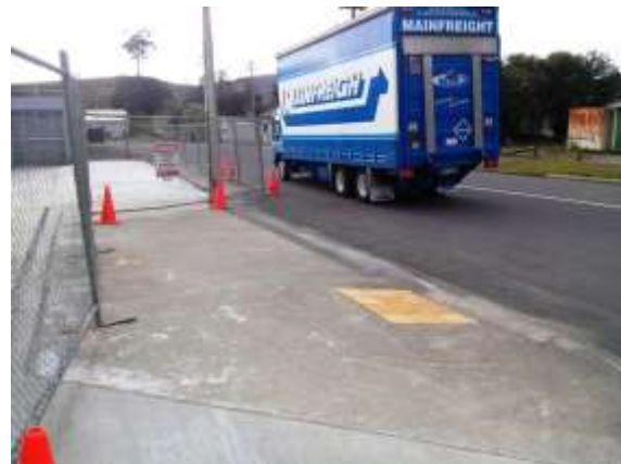
Figure 39: Temporary Traffic Management on Victoria Street
