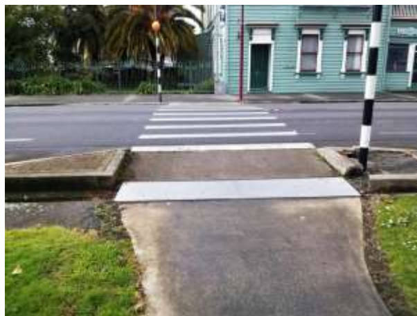
Figure 33: Pedestrian Crossing on SH.2
