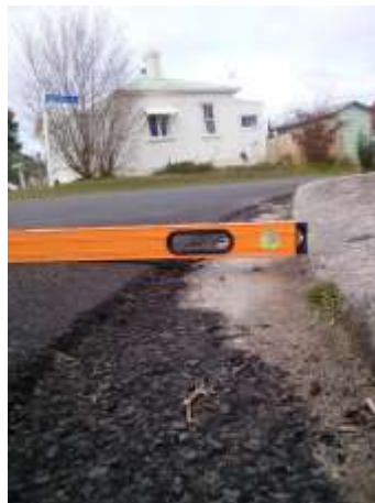
Figure 10: Seal edge join after re-sealing
