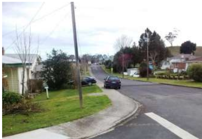
Figure 29: Parking on the footpath at 33 Wood Street
