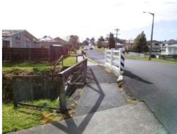
Figure 19: Bridge Barrier on Towers Street
