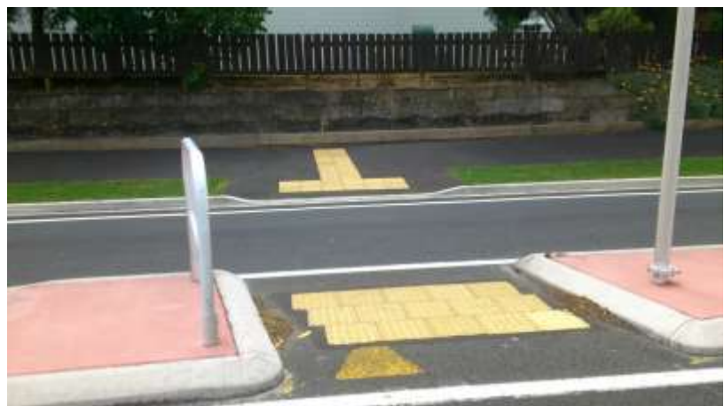
Figure 30: Ideal pedestrian refuge island crossing facility
