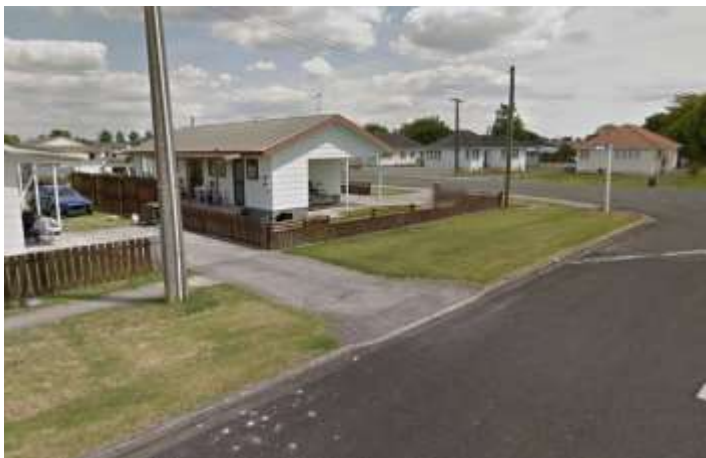
Figure 23: Footpath connection missing at Dearle Street/Opatito Road
