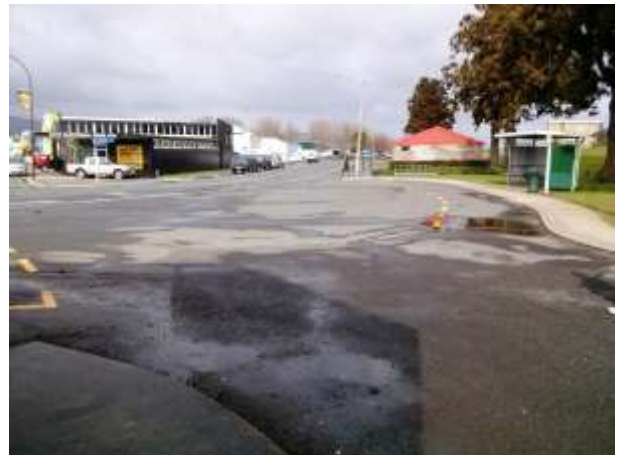
Figure 16: Marshall Street - Entrance to carpark at the intersection with SH.2
