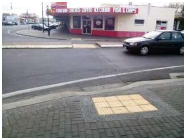
Figure 11: Tactiles at SH.2/SH.26 Intersection
