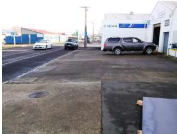
Figure 20: Footpath at Waihi Farm & Industrial Services on SH.25
