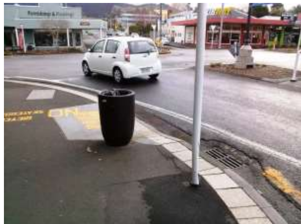
Figure 35: Rubbish bin limiting sight visibility at SH.2/Seddon Street
