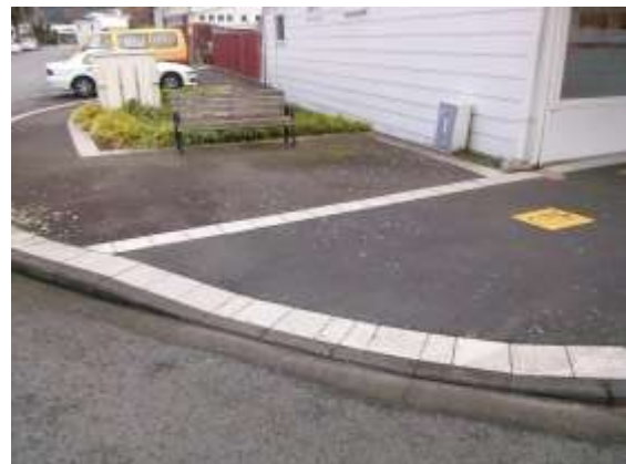
Figure 10: Lip Kerb at SH.2/School Lane
