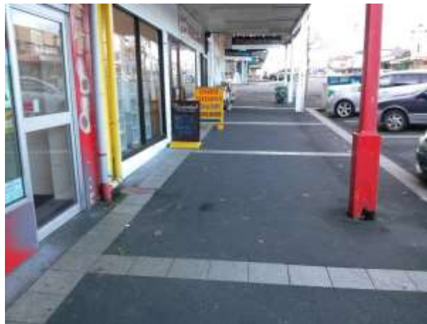
Figure 23: Excellent footpath surface on Seddon Street
