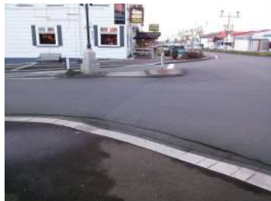
Figure 12: Lip kerb at Seddon Street/Mueller Street Intersection.
