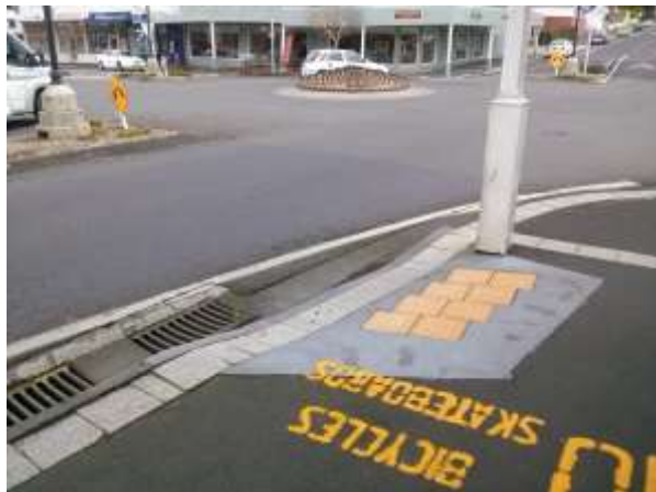
Figure 14: Tactiles at SH.2/Seddon Street Roundabout
