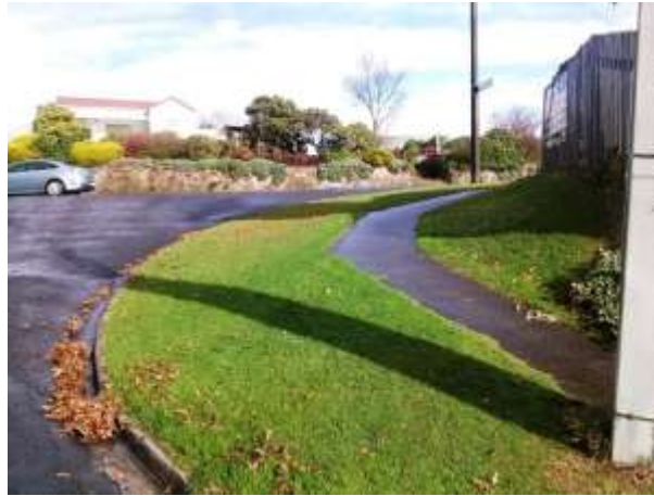
Figure 24: Steep berm at SH.2/Gilmour Street Intersection.
