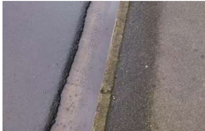
Figure 13: Seal edge join after re-sealing
