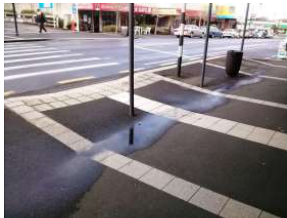
Figure 37: Verandah support at SH.2 pedestrian crossing near Kenny Street
